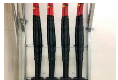
24CSJA-S cold-shrinkable straight joint
