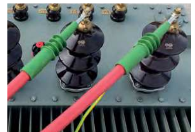
AIP20 as a transformer connection
